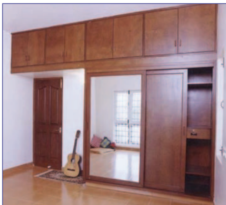
Cabinet made of jute core board.
